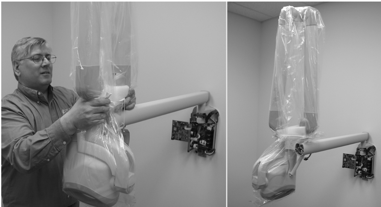
Figure 20 Installing the Articulating Arm and Tubehead Assembly
